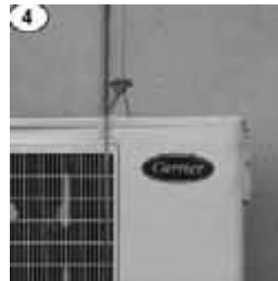
Step 4: Throw the steel wire down from the crosspiece, pass it under the machine and hang it on the wire. Lift the machine some centimeters to balance it before raising it up.
